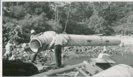
1980-015-258c Construction of Arbutus Outfall 1955
